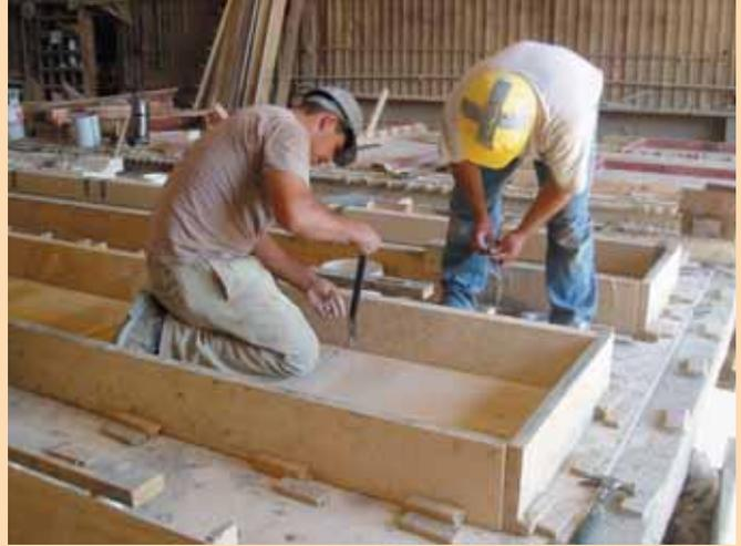
Precasting the concrete panels for the building’s bands called for precise work; the tolerance of  $\pm \frac{1}{64}$ " is twice as small as what’s often used. (Photo courtesy Enterprise Precast)
