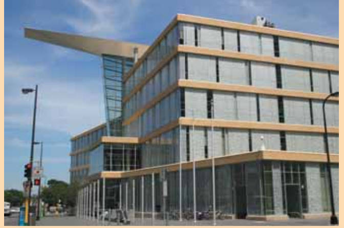
(Above) The native Minnesota Kasota stone makes up the bands that separate the floors of the library building. (Lower left) The stacked stone outside the library effectively covers a rise in elevation. (Photos by Tim Heitman)
