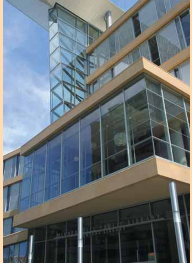
The Minnesota Kasota stone panels, according to one of the building's architects, "provide a visual contrast between the solid and the transparent." (Photo by Tim Heitman)
